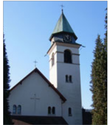
Church with AFILS system installed
