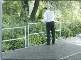
Guard rail (3-sides) as protection against falling
