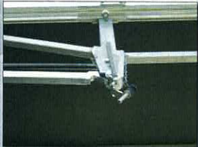
Braces secure the roof
